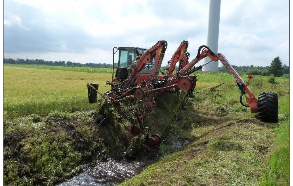
Opening the ditch with expandable ditch & bank rake
