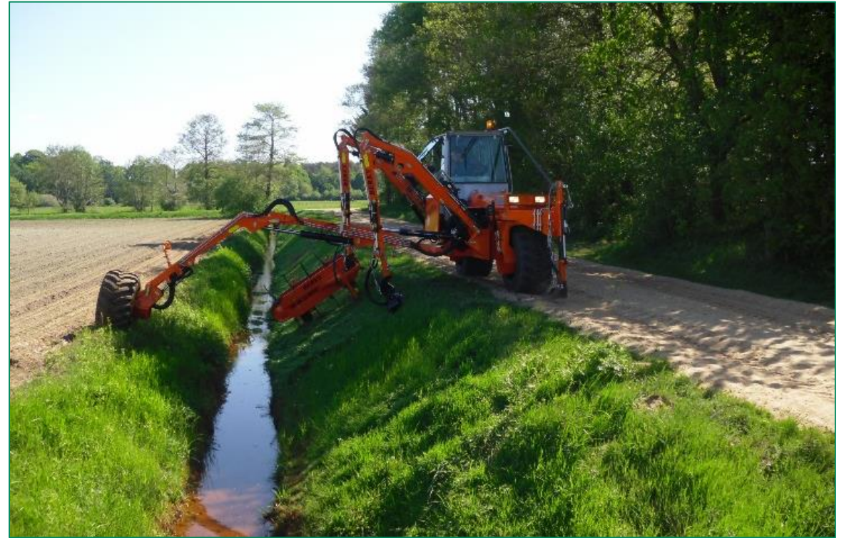
Stabilizer can reach to opposite side of the ditch
