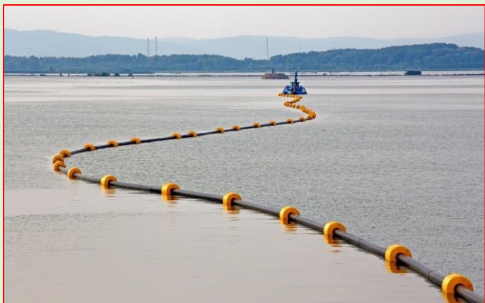
⚙ LONG DISTANCE PIPE LINE DREDGING
