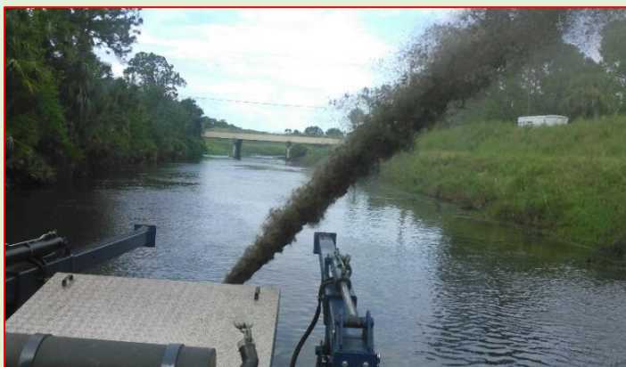
⚙ SIDE CASTING SYSTEM OF SPOILS & MUD ON LAKE SHORES, RIVERS & CANALS
